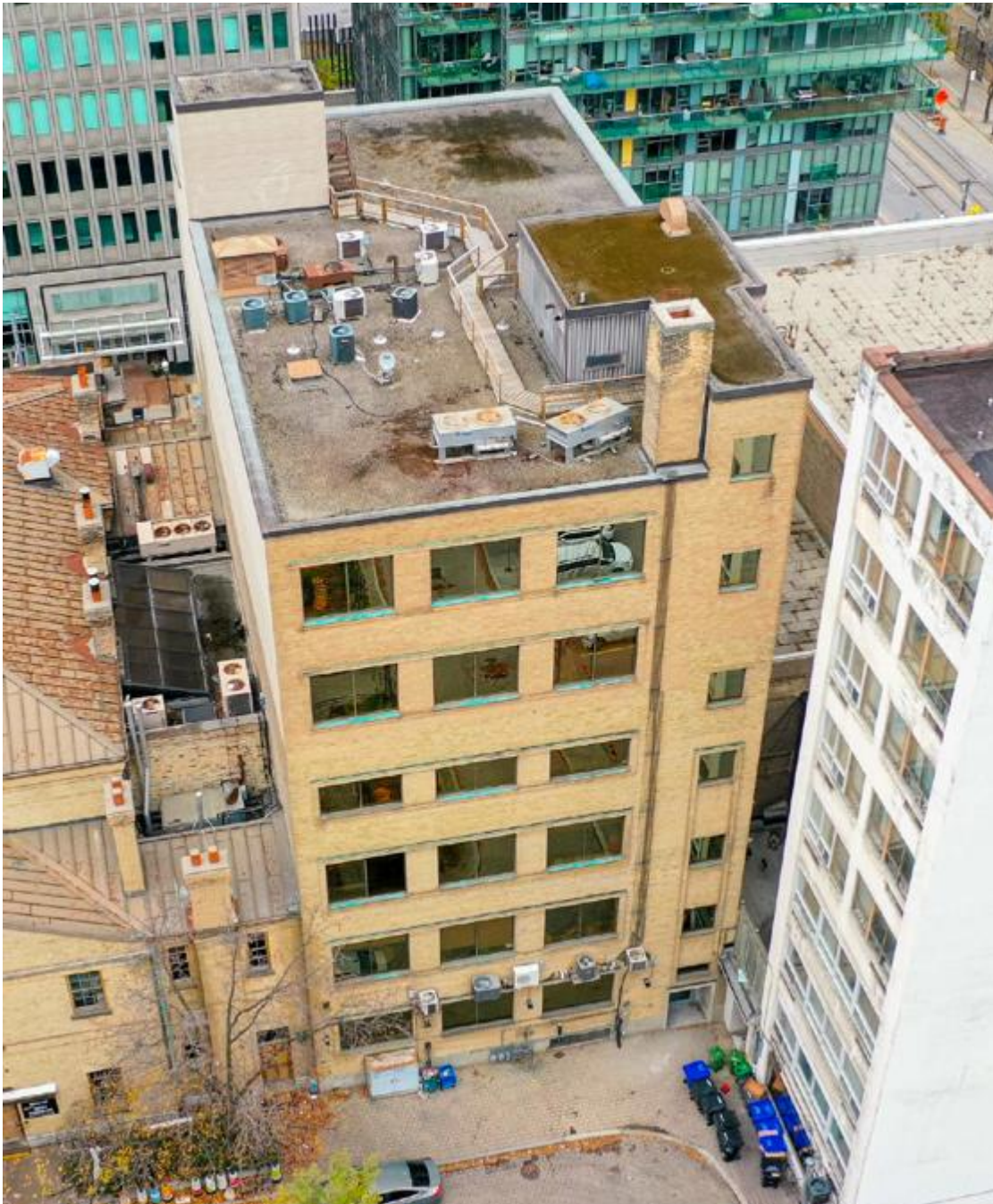
Court Street view
